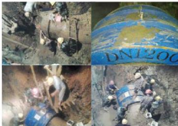
To Repair the socket part of DN1200 cement pipe burst in Hunan Water Group, they use Zhuhong Customized Non-Standard Socket Pipe Repair Clamp efficiently.
