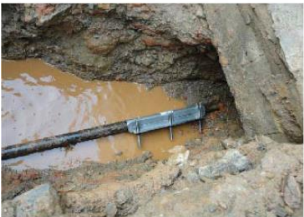
5.For the severely corrosive DN50 water supply pipe of Dalian Insulator Group, Zhuhong Repair Clamp repairs the leakage in very short time.
