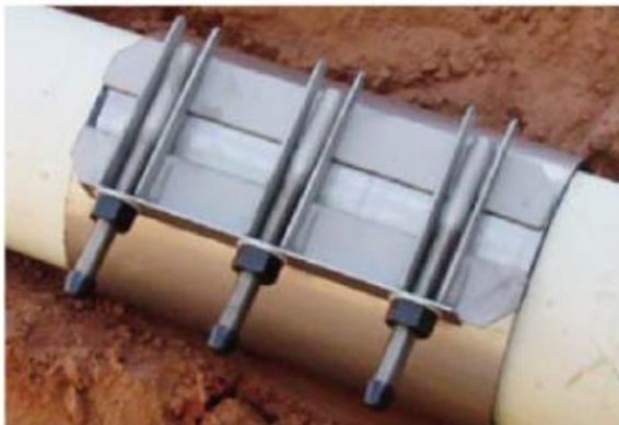
Step4 Use a tension wrench to sequentially tighten the studs to the recommended tension specified on the clamp.
