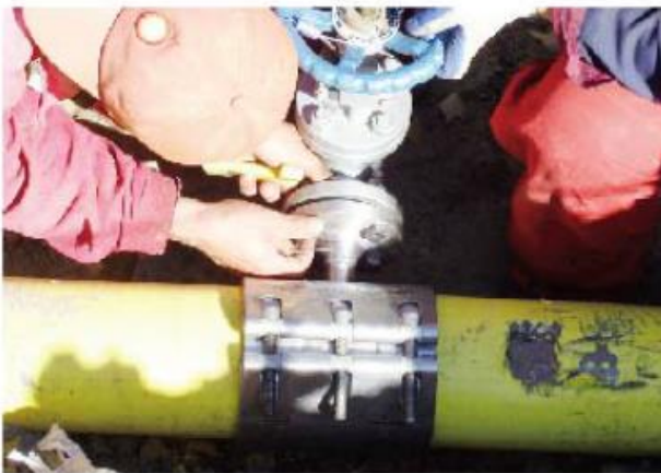
For DN150 pipe with DN20 branch, Daqing Oilfield adopts Zhuhong Multi-Function Tee Clamp to install with hoisting and sealing on nonstop pressured pipeline.
