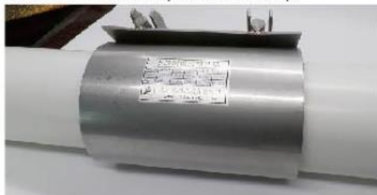
Step5 Installation Finished.
