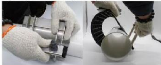
Step2 Wrap the clamp around the pipe, take note to make the overlap of the rubber away from the leak point.
